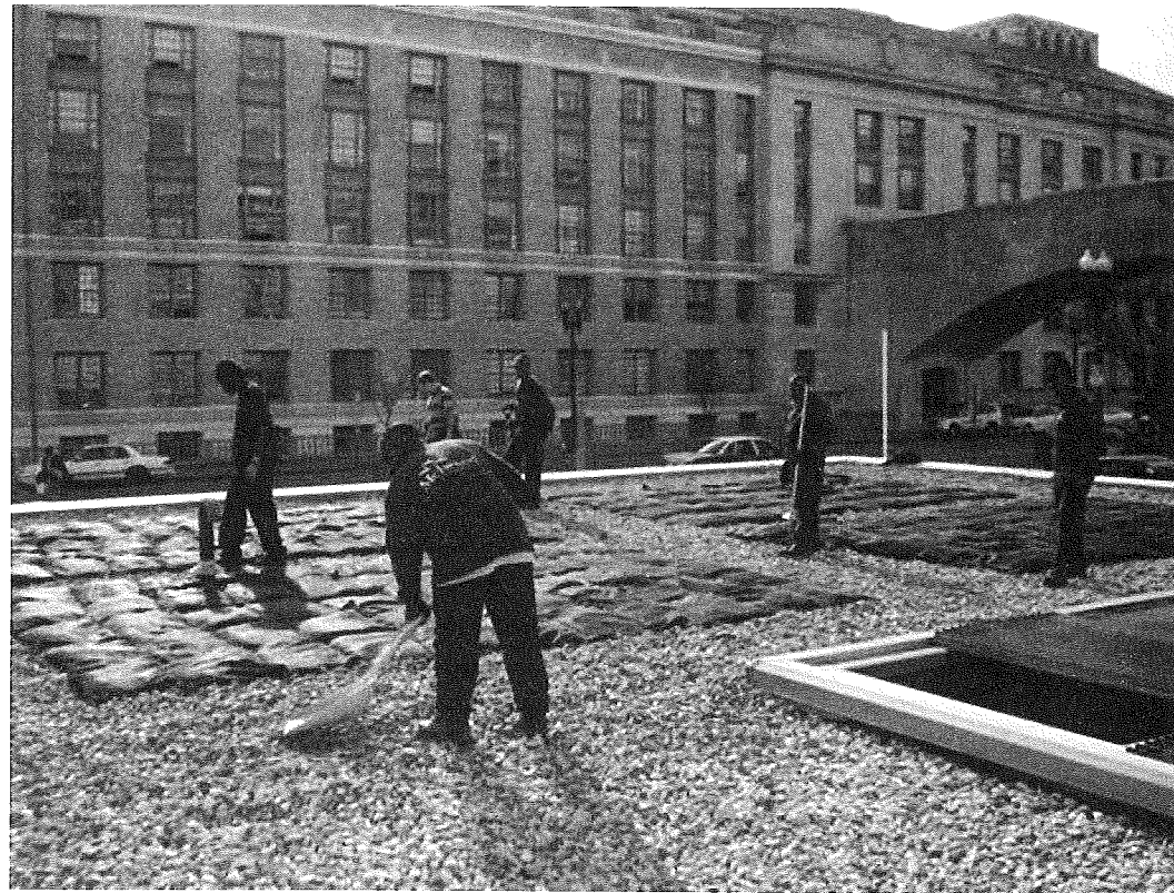
Figure 12.5 Installation of a green roof at the USDA in Washington, DC.
